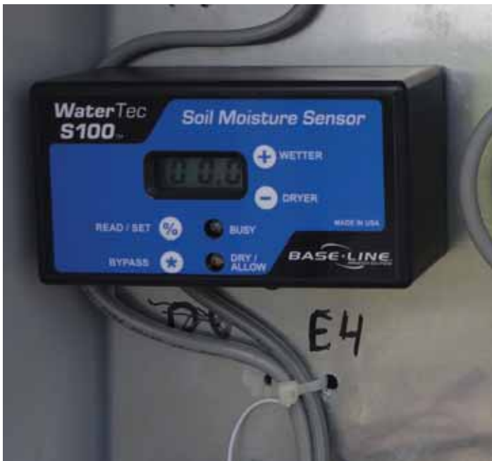
Figure 2. An example of a soil moisture sensor control panel. Credits: Michael Gutierrez, UF/IFAS
